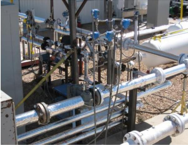
A bank of coriolis meters that measure liquid hydrocarbons and water.
