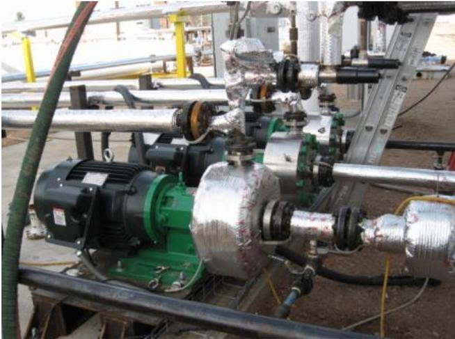
Photo by Magnatex Pumps, Inc. A magnetically driven centrifugal pump used in CL-WGTF.
